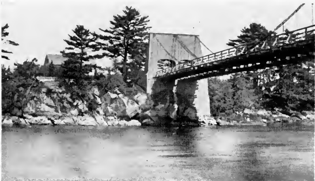
DEER ISLAND AND CHAIN BRIDGE
